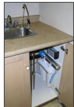
Typical Installation for drinking water under the sink
